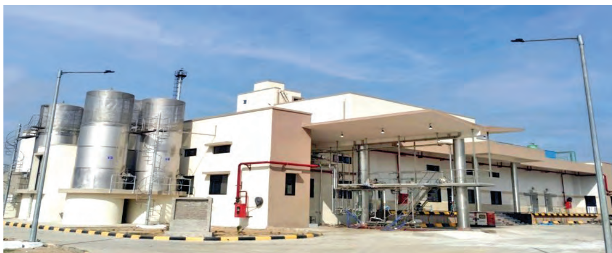
New dairy plant at Palamu, Jharkhand
