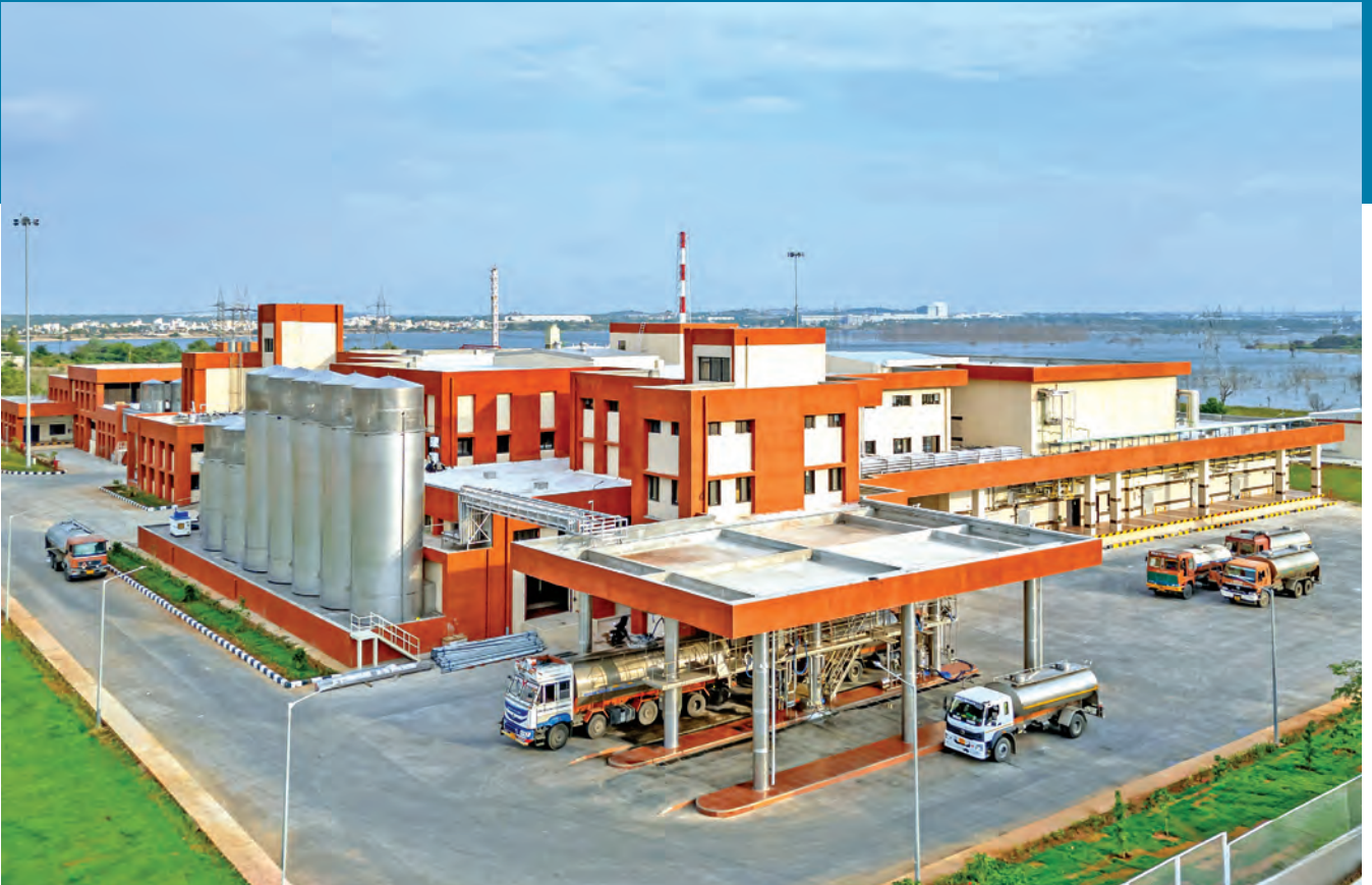
State-of-the-art Mega Dairy Plant, Hyderabad, Telangana
