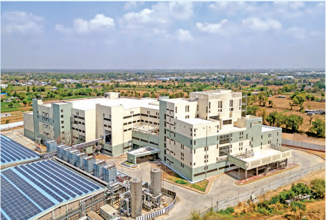
Cheese Plant of Sabar Dairy, Himmatnagar, Gujarat
