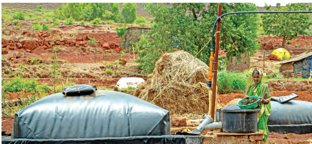
Biogas plant installed under "Gobar Se Samruddhi" Biogas Programme at Kolhapur, Maharashtra
