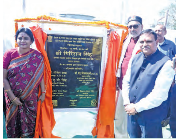
Shri Giriraj Singh, Hon'ble Minister of Rural Development & Panchayati Raj laying the foundation stone for a 100 MTPD capacity dung-based biogas plant at Barauni Dairy
