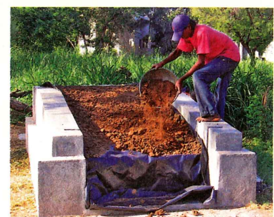
Sealing of silo
